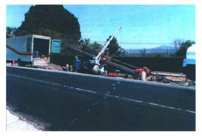
Horizontal directional drilling was used on pot. dons of the project where other construction methods were impractical or impossible. Another contractor had tried unsuccessfully to make most of the bore completed by Dynamic Cable Construction Cu Dynamic was called in to use its larger equipment with rock drilling capabilities.
